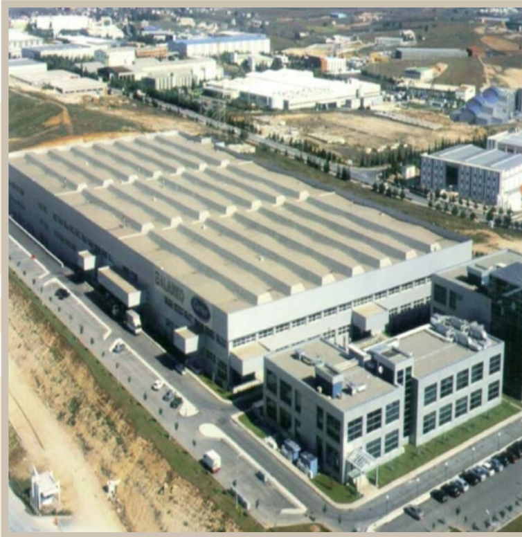
Alarko Carrier Production Plant – Istanbul, Turkey
